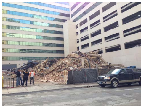
Remains of the Thomas building after demolition.
