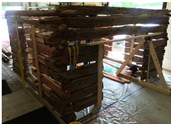
The recent stabilization of the cabin provided further insights into the craft of the cabin's construction as the original wood pegs and hand hewn logs with notched and pegged connections at wall/roof conditions were revealed..... these are remarkable, well-crafted construction techniques utilized in this log building that was built without the use of nails (or other metals)."
